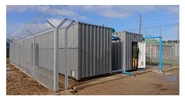
The packaged potable water treatment plant (PWTP 050) will treat 54m<sup>3</sup> of water per hour, which is fed into the municipality's bulk water supply. Fabricated in 12 weeks at Veolia's Water Techno Packages facility in Sebenza, Johannesburg, the plug-and-play PWTP supplies the treatment of the borehole water to SANS 241 standards.
