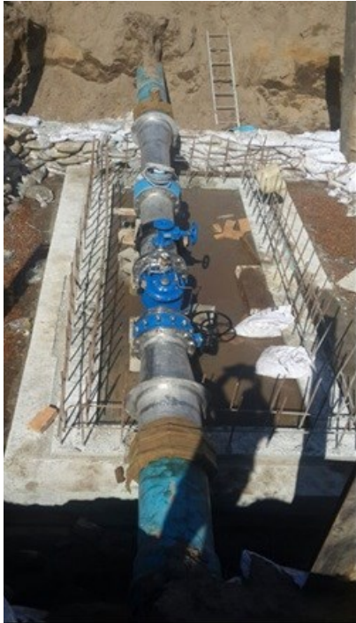
300mmØ bulk water connection installation for Pearl Valley, Paarl
