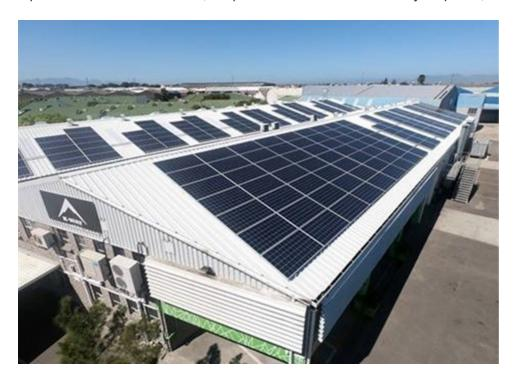
According to K-Way, on the day following installation 200 kilograms of carbon dioxide were saved, despite it being a cloudy winter's day. The 83kWp Solar PV system harnesses the sun's energy to power the factory and produces 125,000-kilowatt hours per year to deliver financial savings whilst reducing the factory's environmental impact.
