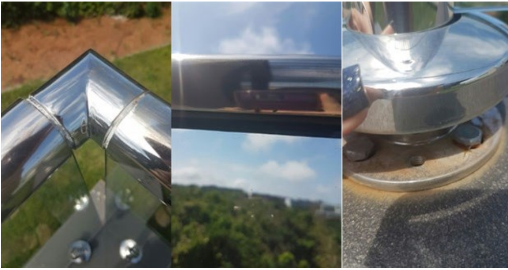
Example of sub-standard stainless steel balustrade installation in KwaZulu-Natal.
