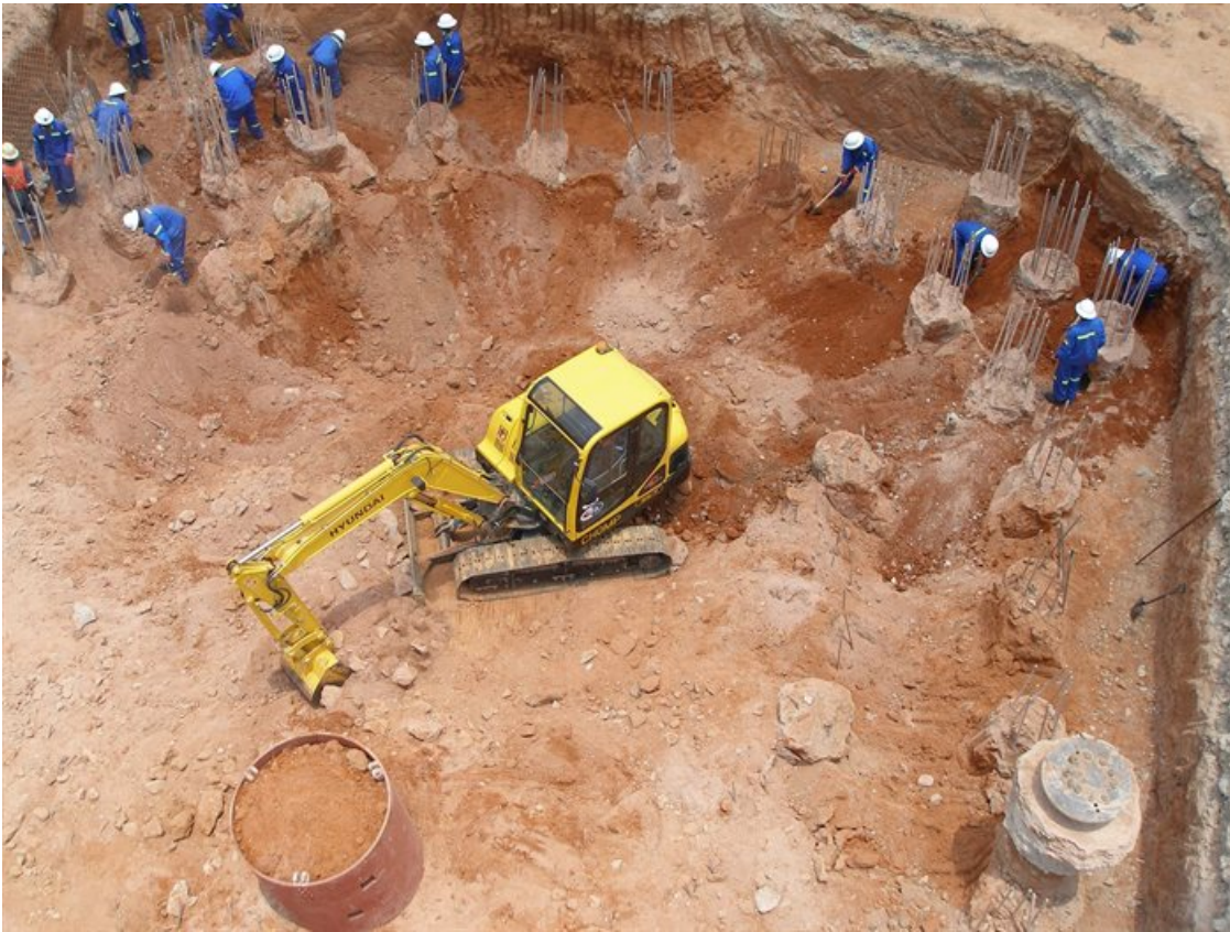
A detailed ground assessment ensures that shallow vertical cuts will remain stable. (Image: SRK Consulting)
