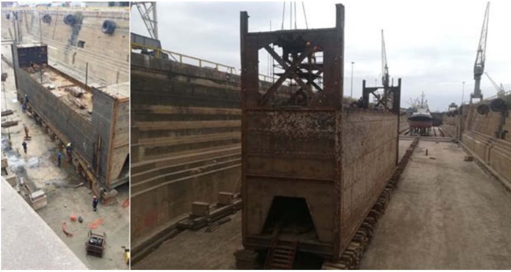
Removal of the air chamber (left) and sealing faces (right) on the Prince Edward Graving Dock's inner caisson.
