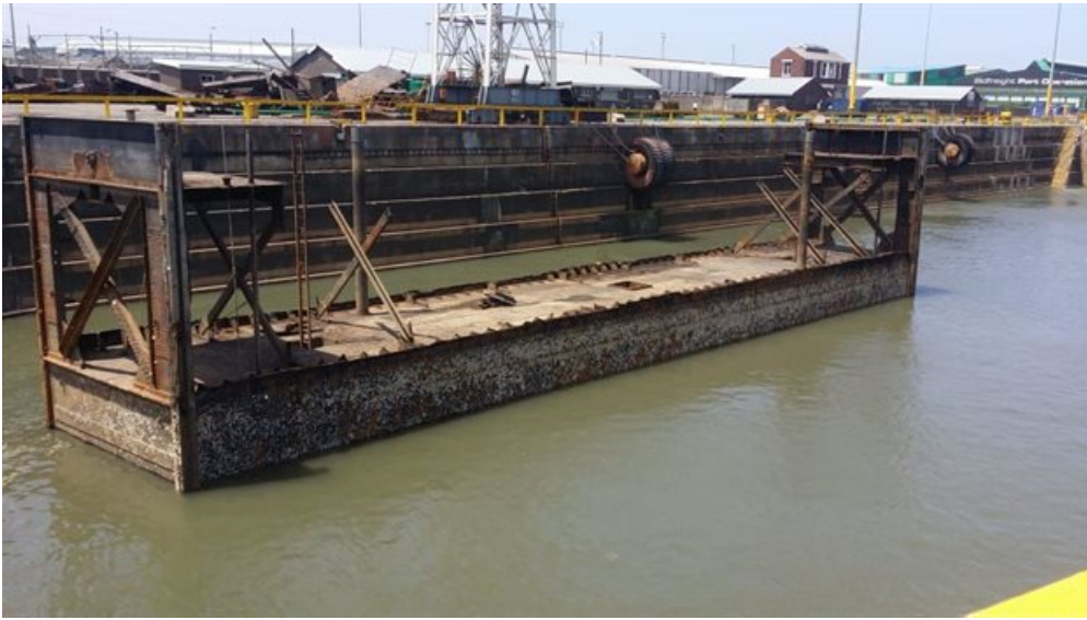
The Prince Edward Graving Dock's inner caisson had deck A and B removed and cut up for scrap.
