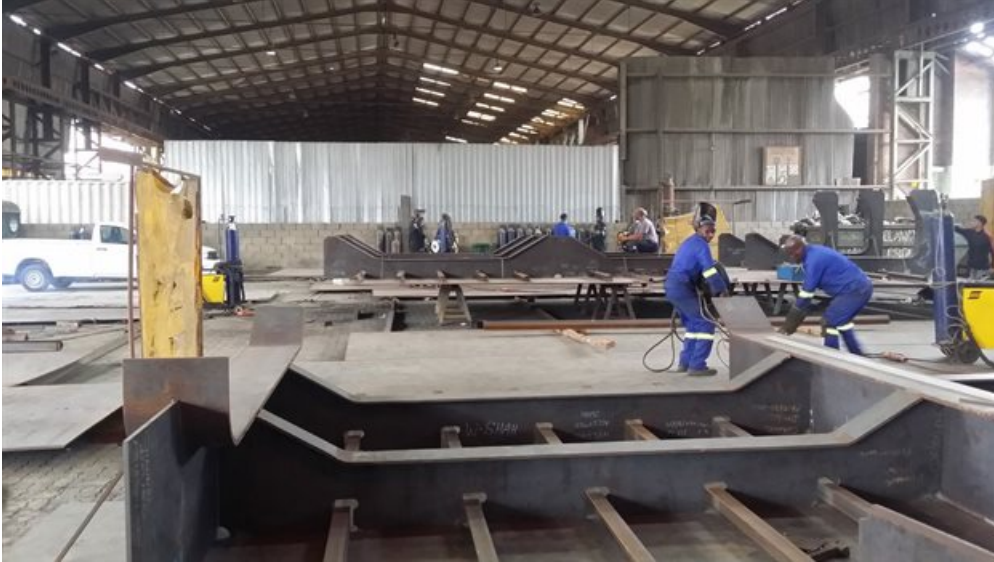
The rehabilitation of the Prince Edward Graving Dock's inner caisson includes major structural design improvements on re-built decks and compartments, which are being built in a controlled environment in an off-site engineering workshop.
