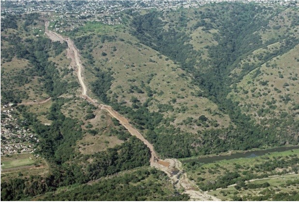
Western Aqueduct pipeline crossing the Umgeni River through the Umgeni Valley. Rehabilitation of environment is still due.
